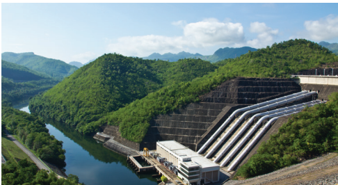
SMALL HYDRO ENERGY
